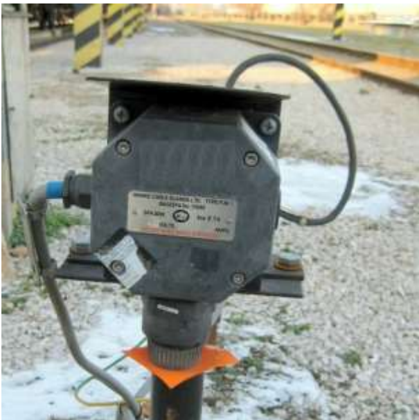
Picture 1 gas detector inhibition with adhesive tape
