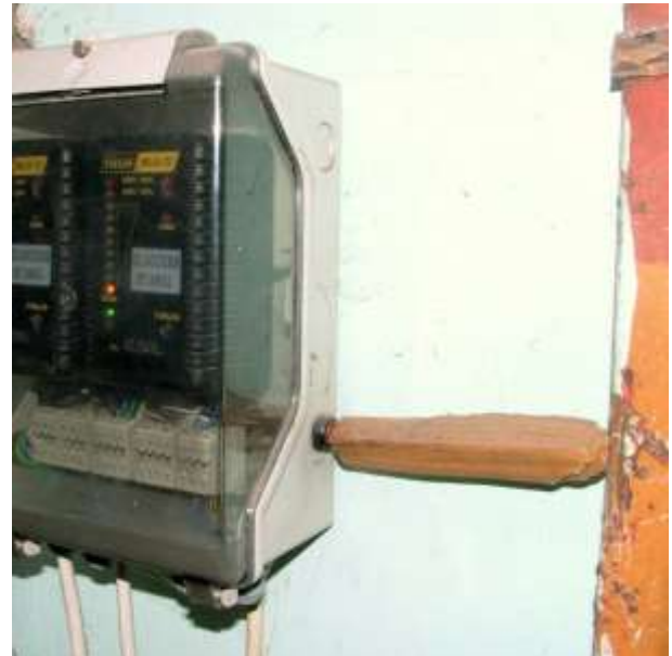
Picture 5b ack. button supported by a piece of wood
