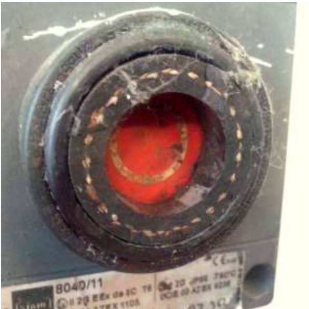
Picture 8 flexible rubber hose insertion
