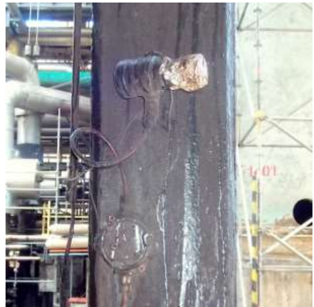
Picture 2 gas detector inhibition with aluminium foil
