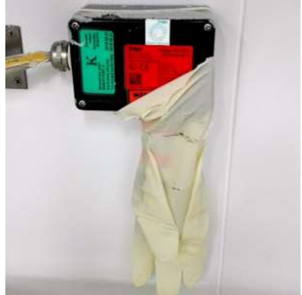
Picture 4 gas detector inhibition with latex gloves
