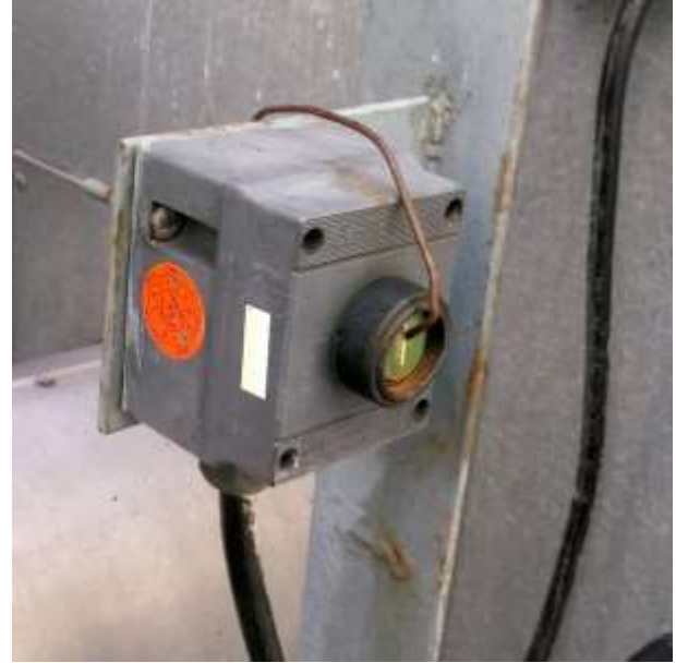
Picture 7 spring steel wire fixing
